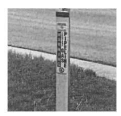
absence of a pipeline marker does not mean that an underground pipeline may not be present.
